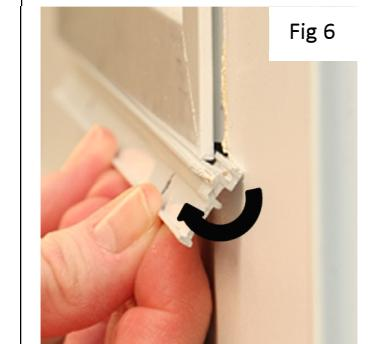
From the outside of the door, remove the pet door frame.
