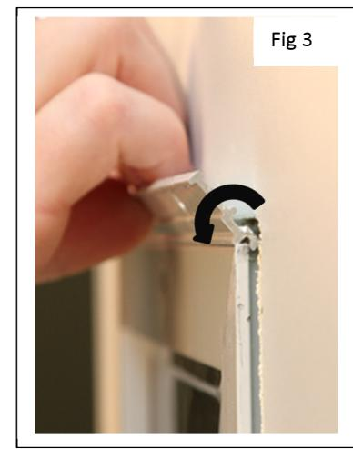
Place a flat screwdriver against the edge of the bottom lock trim (Fig 4). Tap the handle of the screwdriver until it moves the lock trim  $1-1\frac{1}{2}$ " (Fig 5). Tip the lock trim towards you to release the interlocking lip (Fig 6). You may use a screwdriver to pry. Remove and set aside.
